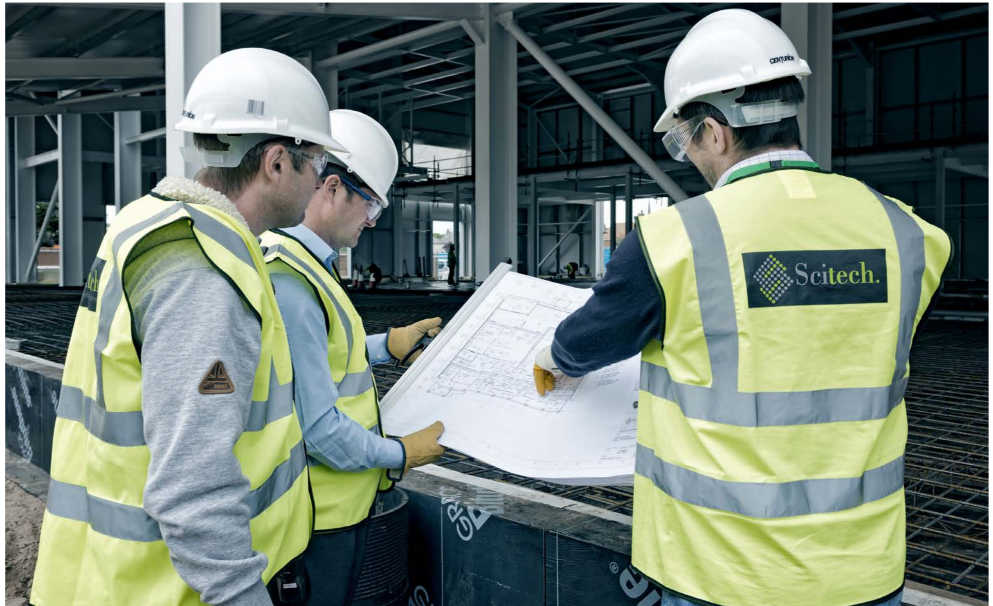
Cleanroom walk on ceiling for blue chip pharmaceutical manufacturer.
